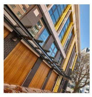
The envelope was designed to protect rightto-light of adjoining owners together with compliance with the London fire plan, and was constructed using composite cladding, masonry and finned rainscreen system.
